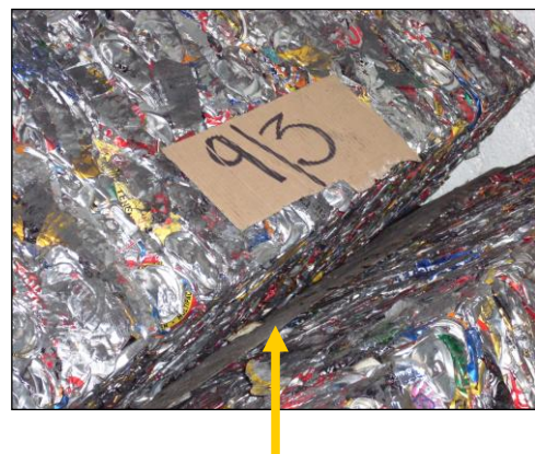
Drain for top layer of bales made from old roofing
